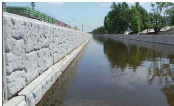
Figure 2: River Retaining Wall
